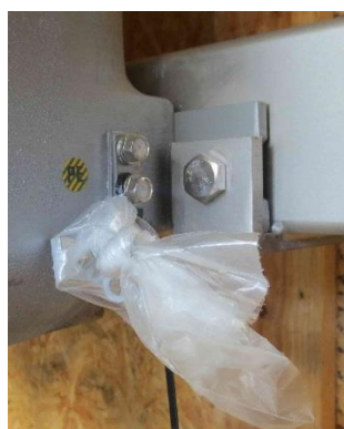
Fig. 6.6: Grounding connector EX-d box
