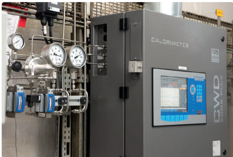
In the calorimeter measuring station the combustion value of the produced process gases is determined using three calorimeters.
